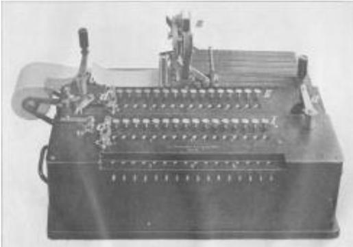
Figure 16: The Hamann Difference Engine. There is no model of the machine nor is the original known to exist any more.<sup>22</sup>
