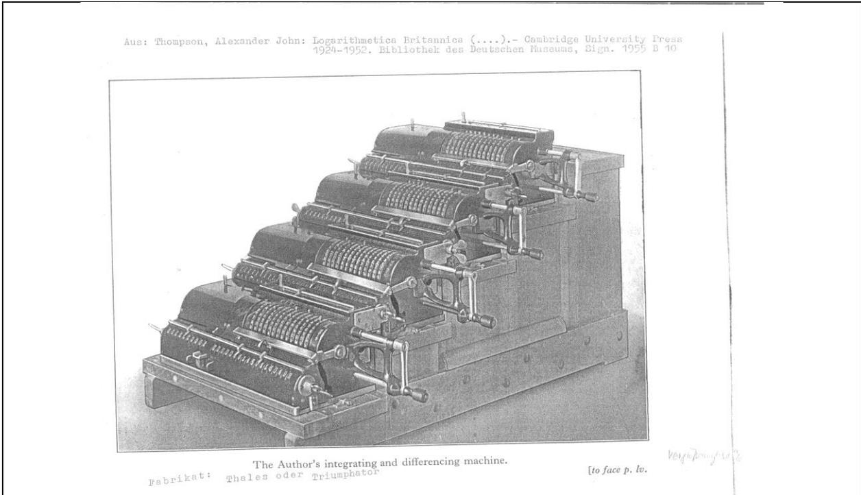
Figure 9: A.J. Thompson’s calculating machine was a combination of 4 Thales/Triumphator machines
